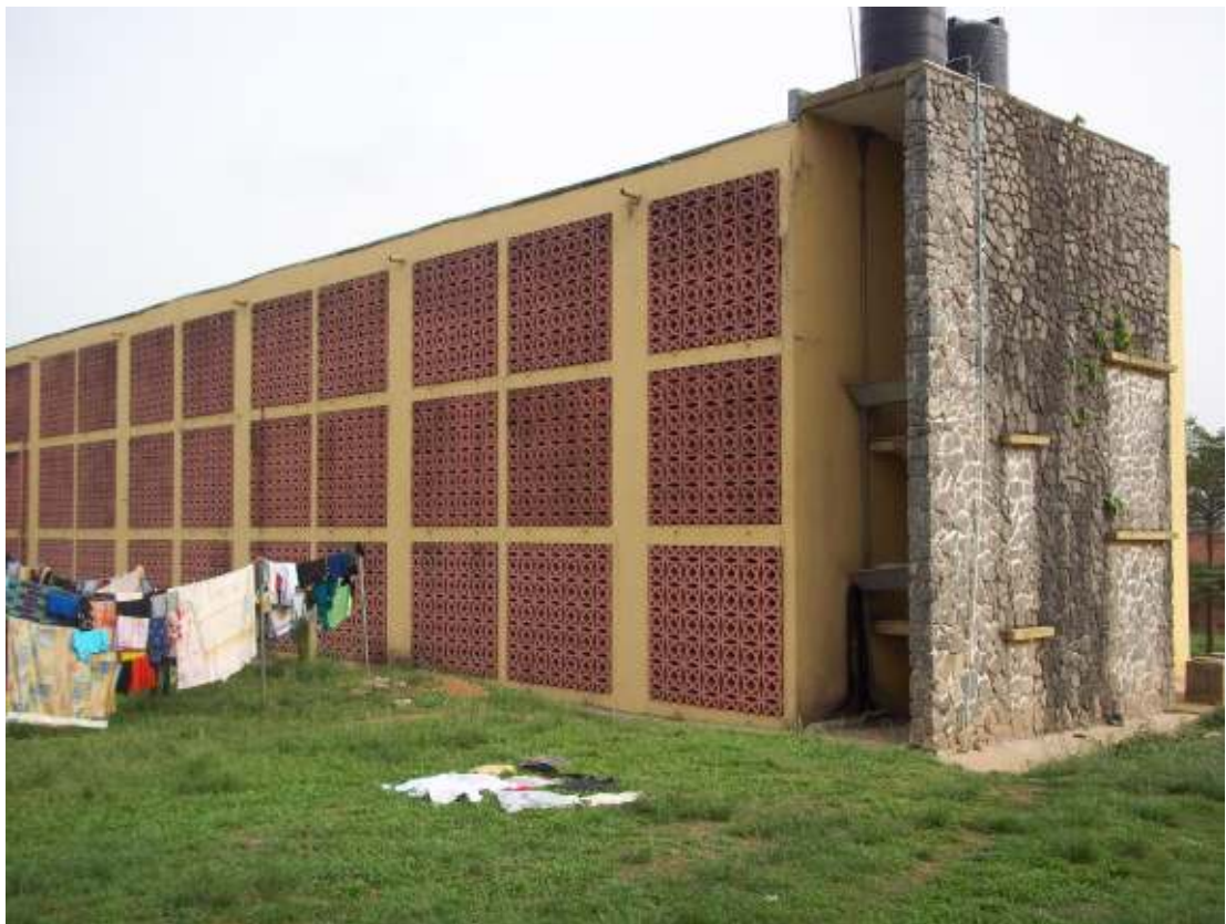
Plate 4: Rear staircase of building slabbed as overhead tank
