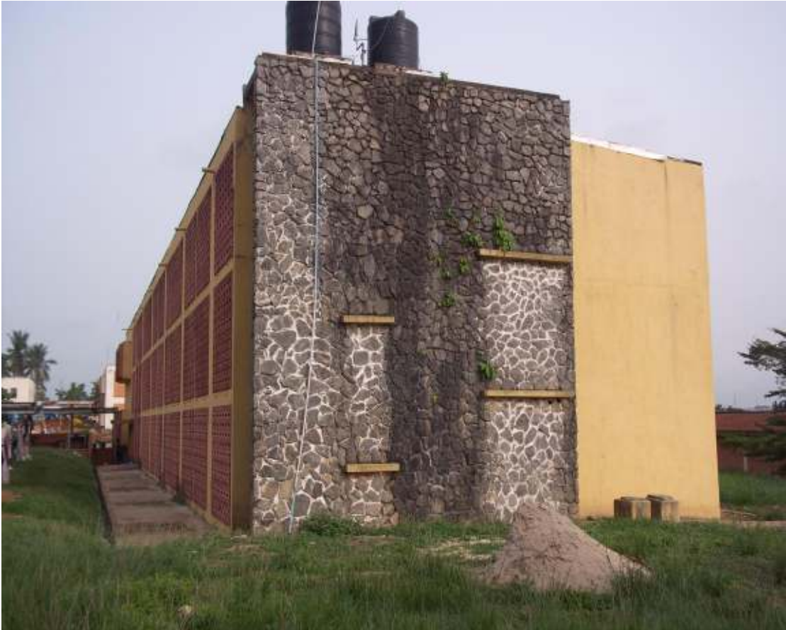
Plate 5: Rear of building
