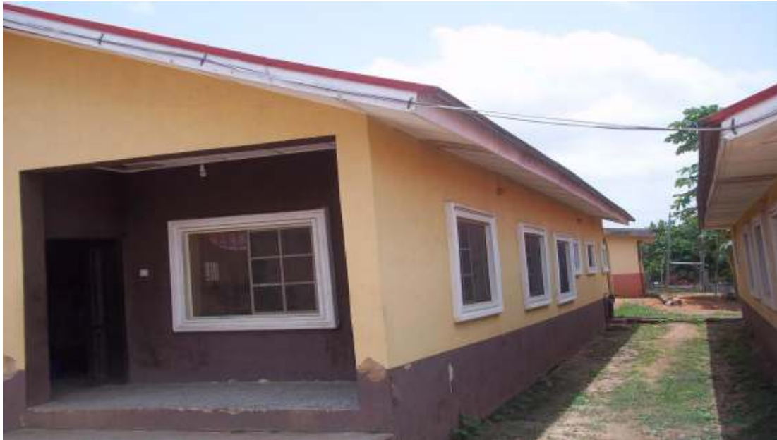
Plate 7: A typical front view of Cafeteria hostel blocks
