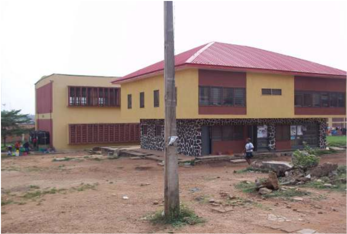
Plate 3: A view of the hostel
