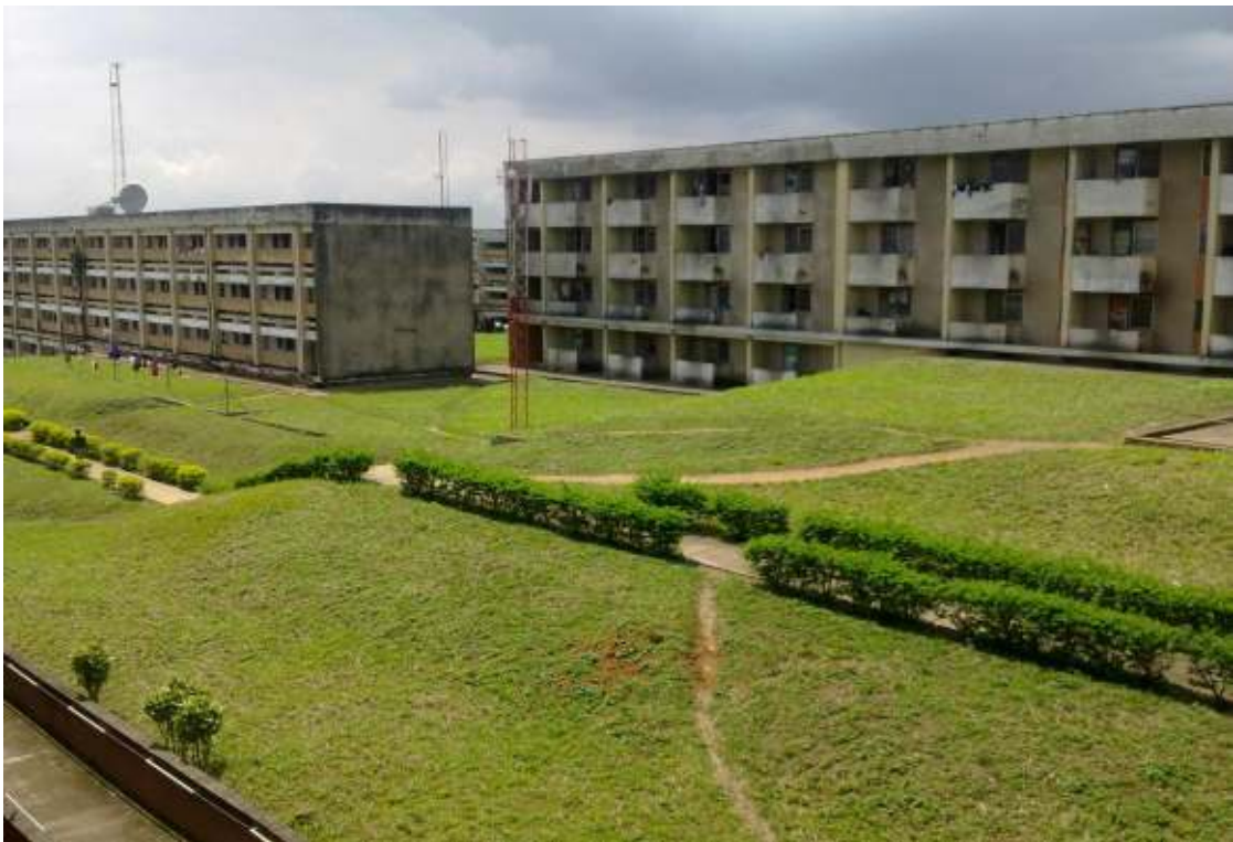
Plate 11: A view of the hostel
