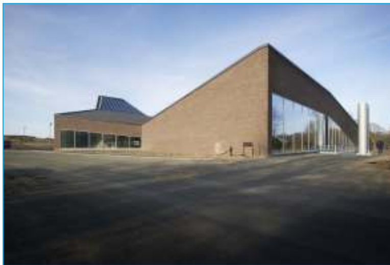
Plate 42: Approach view of the Vandhalla Egmont Rehabilitation Centre.
