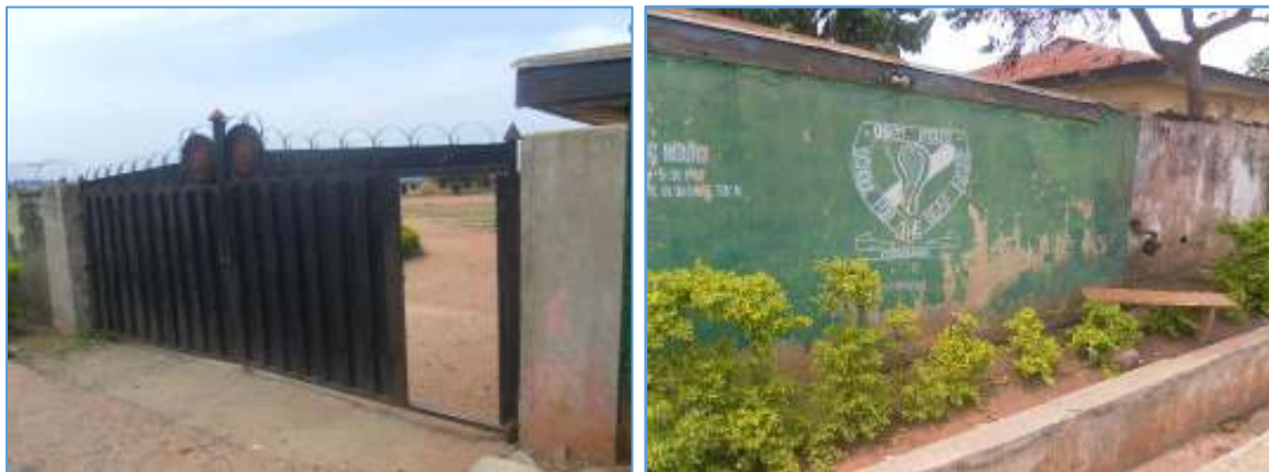
Plate 24: Showing the gate and entrance area.
