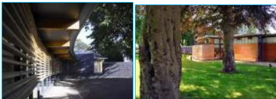
Plate 52: Curved wooden walls and Larch timber boarding.
