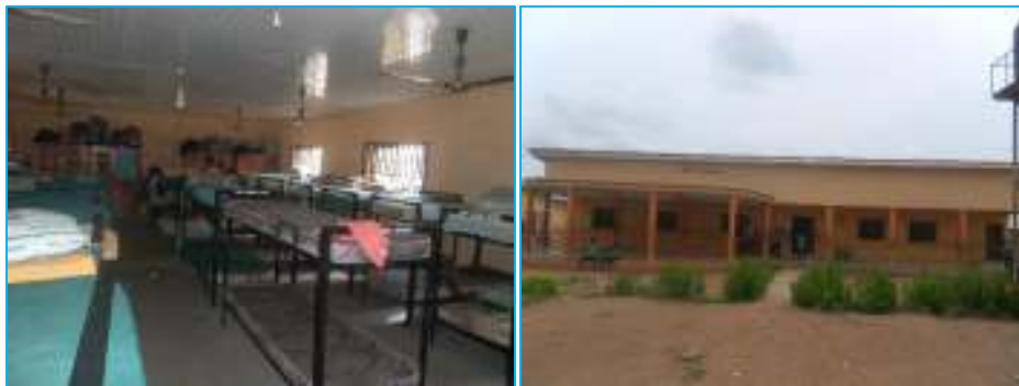
Plate 30: The interior of the hostel and the new hostel respectively.
