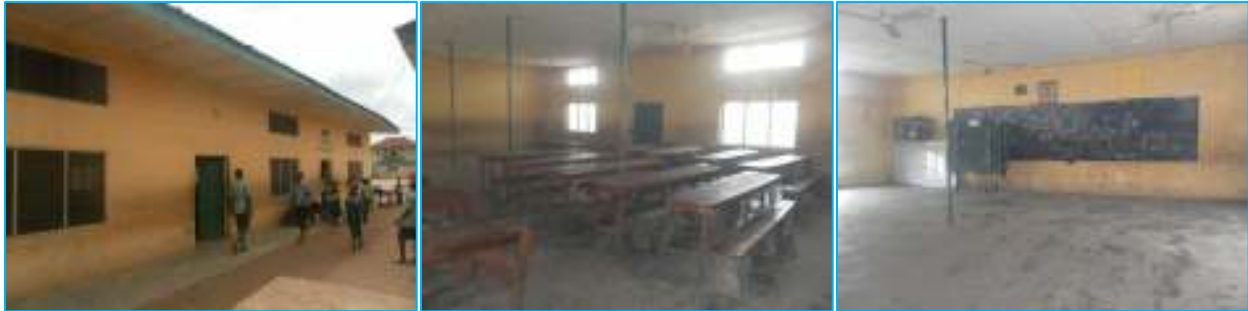
Plate 32: Showing the external and internal views of the building.
