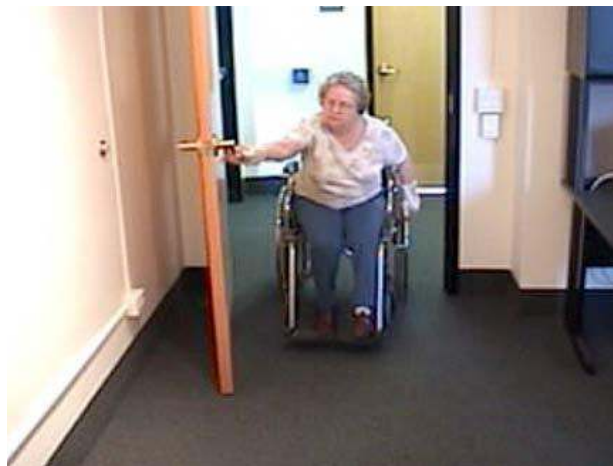
Plate 1: Example of good location of door latch.
