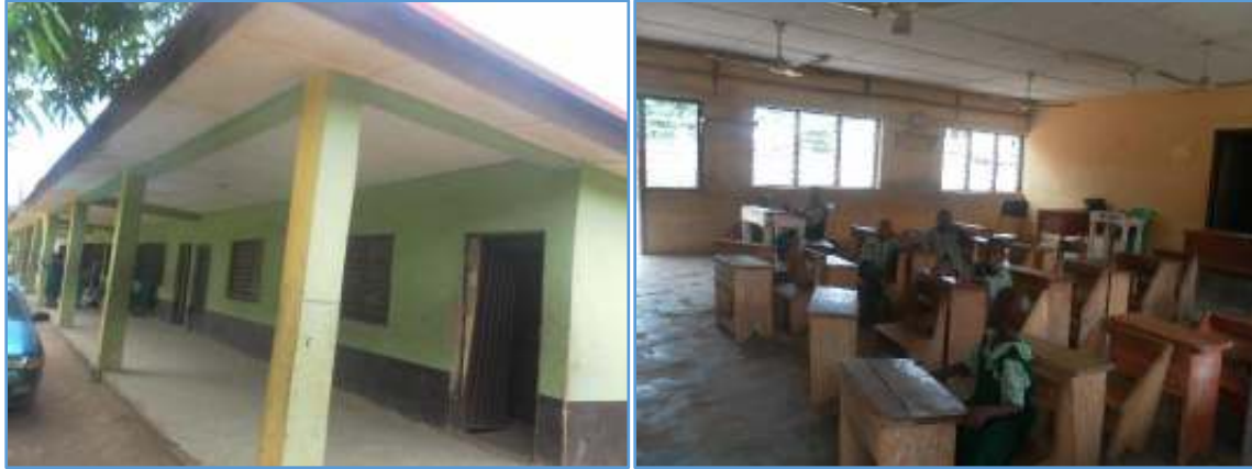
Plate 27: Showing the Block 1 and interior of the class room.
