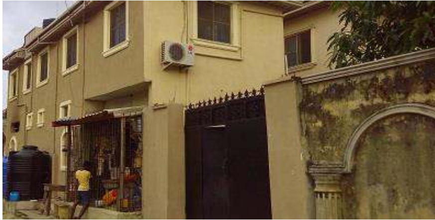
Plate 4.18: External approach of case study 3, showing the nature of the setback space between the approach fence and external drainage
