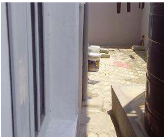
Plate 4.16: sharp sand on side set back space
