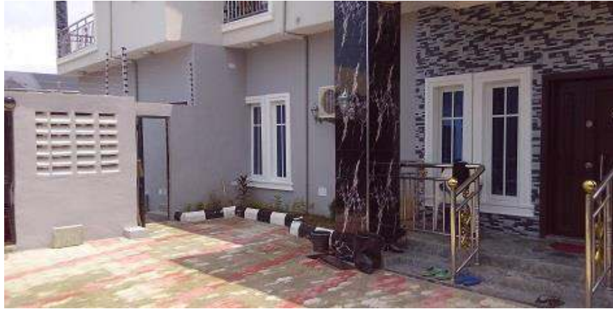
Plate 4.14: State of the setback space between the approach fence and residential building
