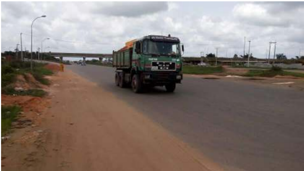
Plate 2.10: Sapele Road End of the Benin By-pass
