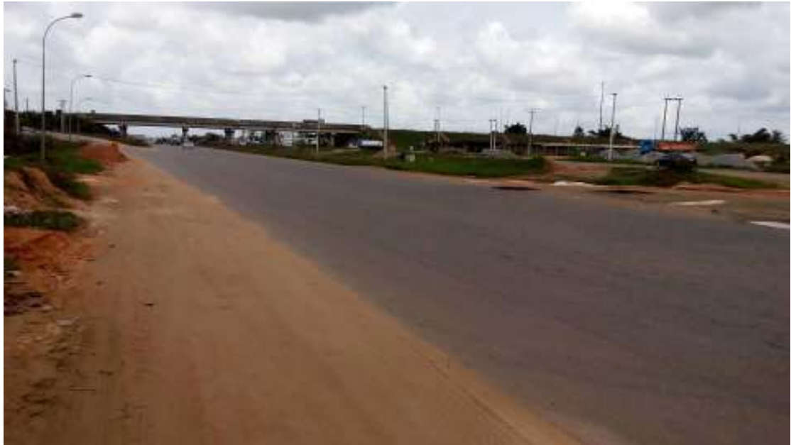
Plate 2.9: Agbor Road End of the Benin By-pass
