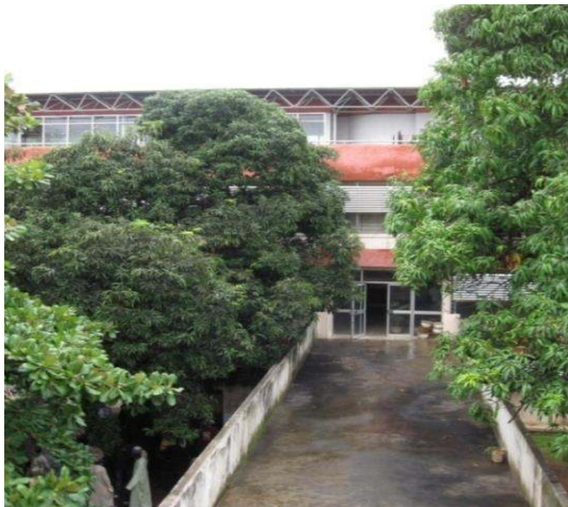
Plate 3.6: Bridged walkway that connects two wings of the department
