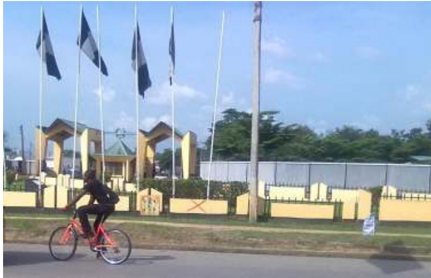
Plate 3.16: View showing the University of Uyo Entrance Gate
