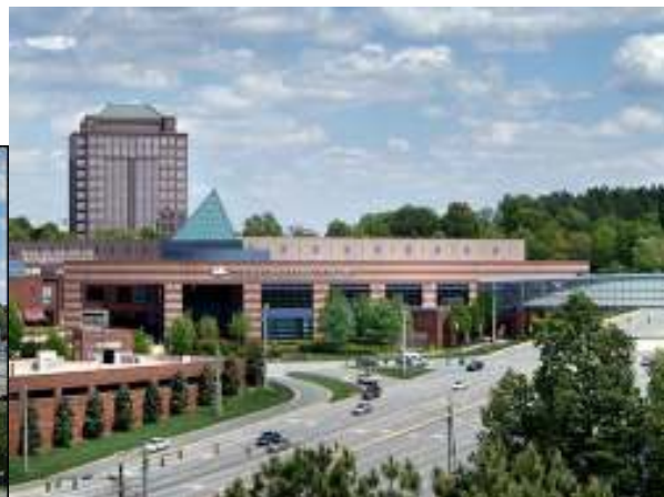
Plate 3.12: Showing the access to the Galleria
