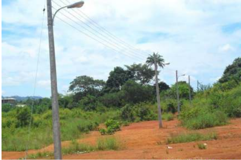
Plate 4.9: Showing the power line adjacent the site
