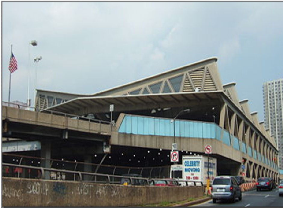
Plate 20: View of the Terminal from the West at 178th St
