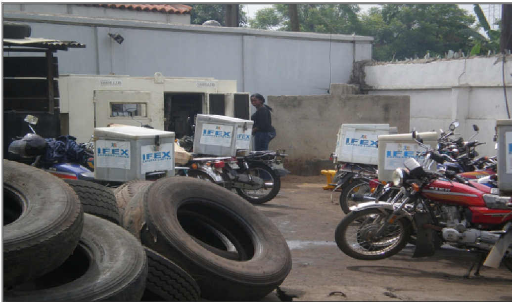
Plate 12: View showing Generator House and IFEX Motor Cycle Yard
