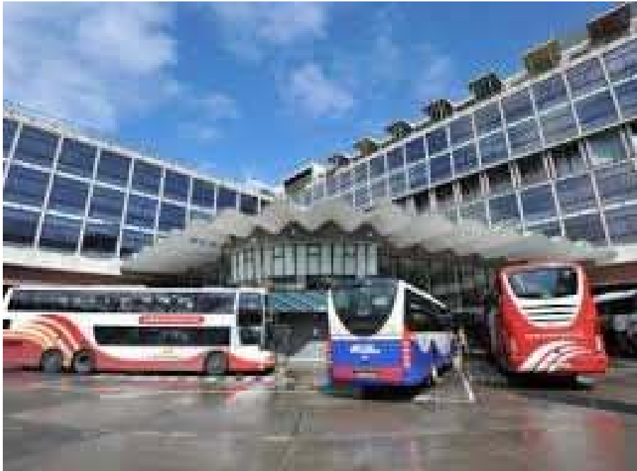
Plate 18: Approach view of Terminal Building
