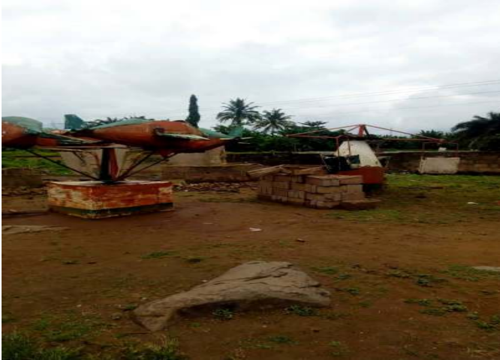
Plate 4.1: Dilapidated recreational facilities at Oyemekun Rocks
