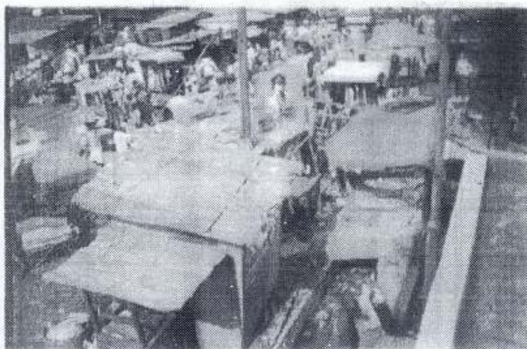
PLATE 1: OYINGBO MARKET, LAGOS. SHOWS THE DETERIORATING CONDITION OF THE MARKET ALONG BORNO WAY.
