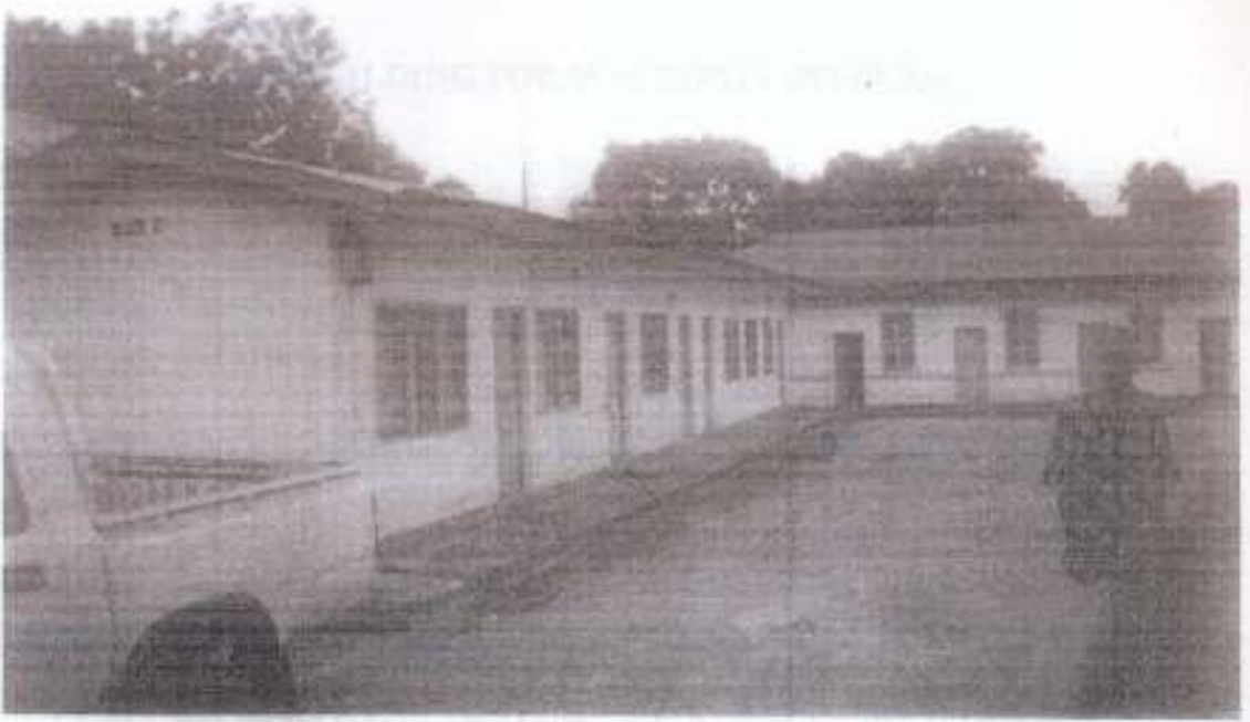
Plate 5: Plate showing the scattered buildings around the Headquarters
