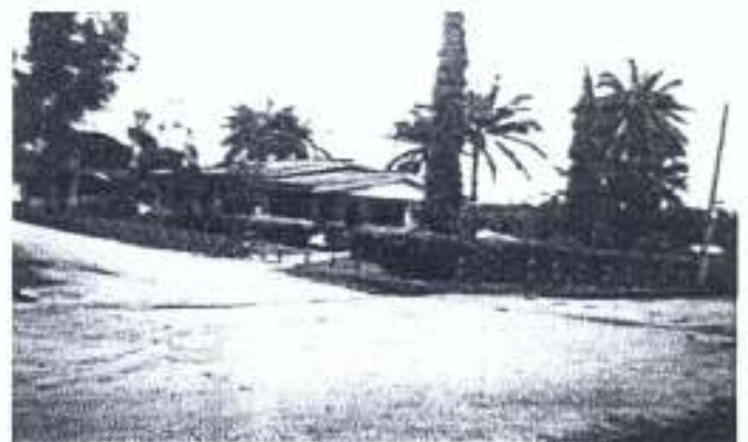
PLATE 14 Showing the Administrative Building at the Camp
