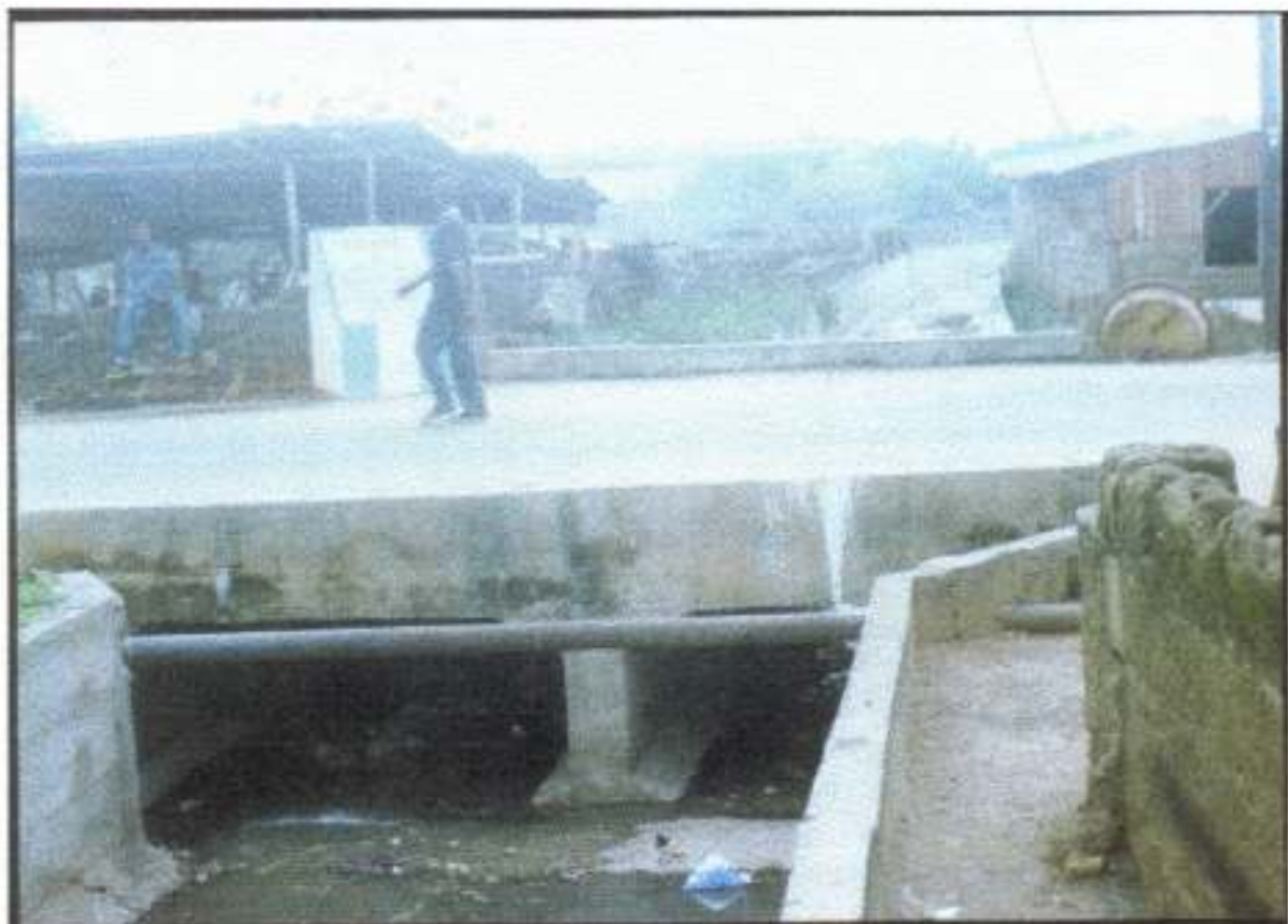
Plate 1: PTF Constructed Drainage and Culvert
