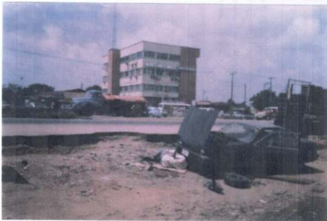
PLATE 3.4: WEMA BANK ZONAL HEADQUARTERS, ABULE-EGBA LAGOS SOURCE: FIELD SURVEY
