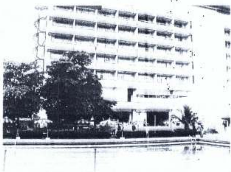
Plate 4.3b: Pool side View of Premier Hotel, Ibadan
