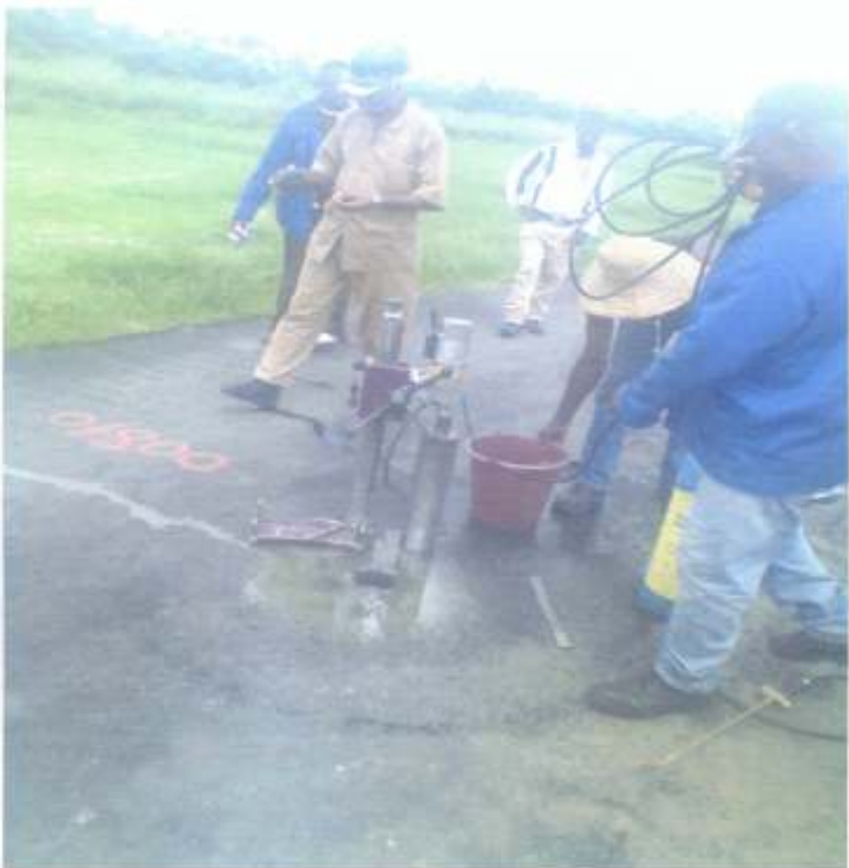
CORING TEST IN PROGRESS
