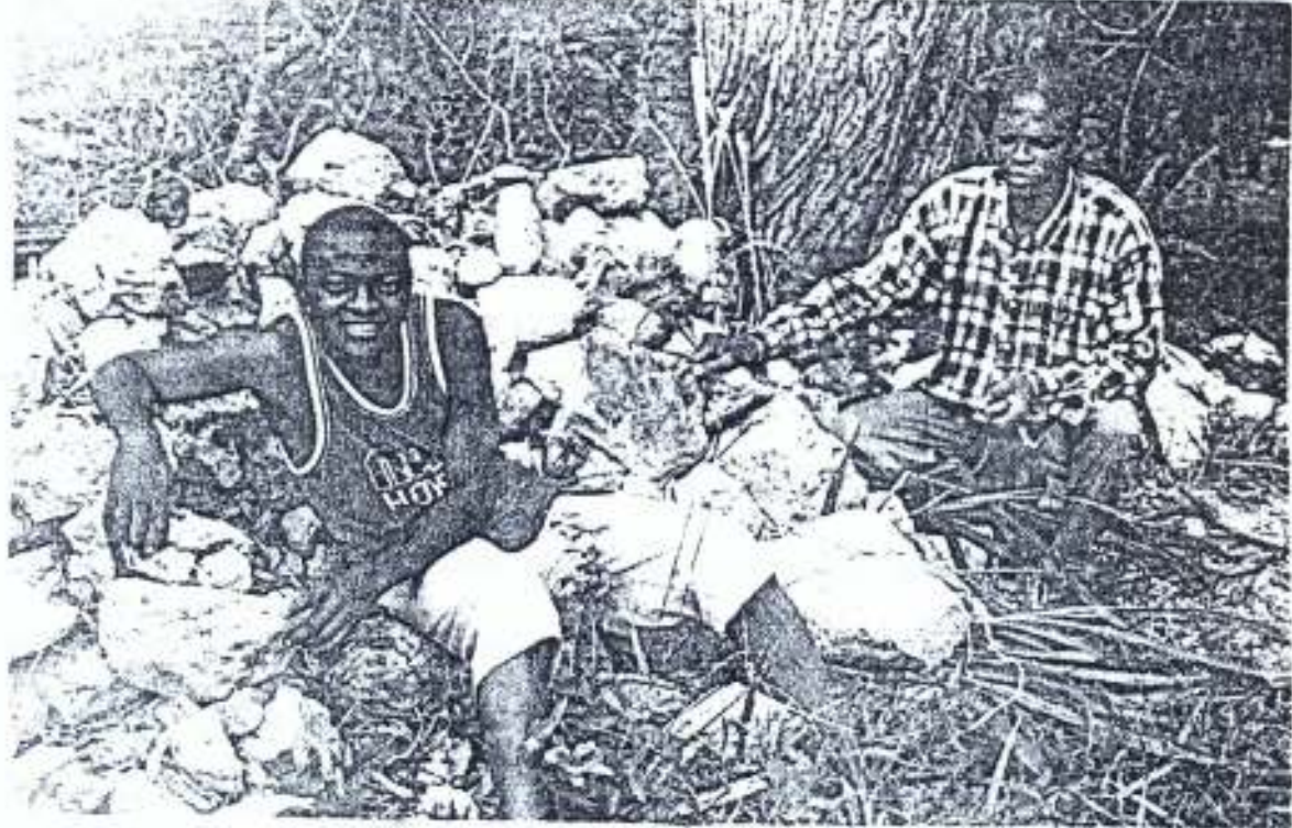
Plate 1: Demolished Concrete Rubbles
