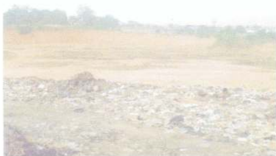
Plate 3.2 : Landfill Pit without sealant, prepared to receive waste.
