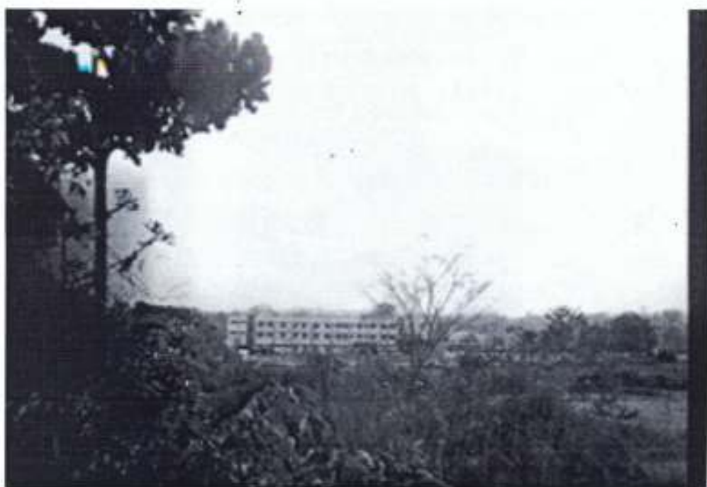
PLATE 3D VIEW OF THE PRESENT ACADEMIC AREA FROM THE TOP OF THE RIDGE. ENGINEERING BUILDING IN THE DISTANCE.
