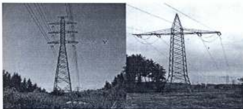
Fig 2.2 330KV and 132kV Electricity Transmission Tower
