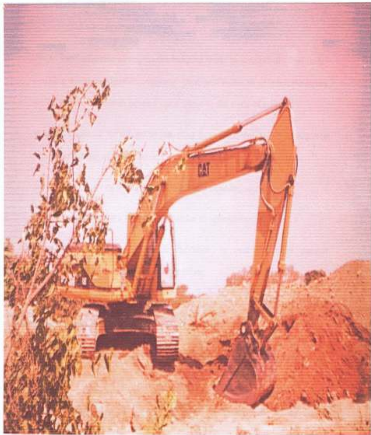
Plate 3.3: Overburden Removal in Azara
