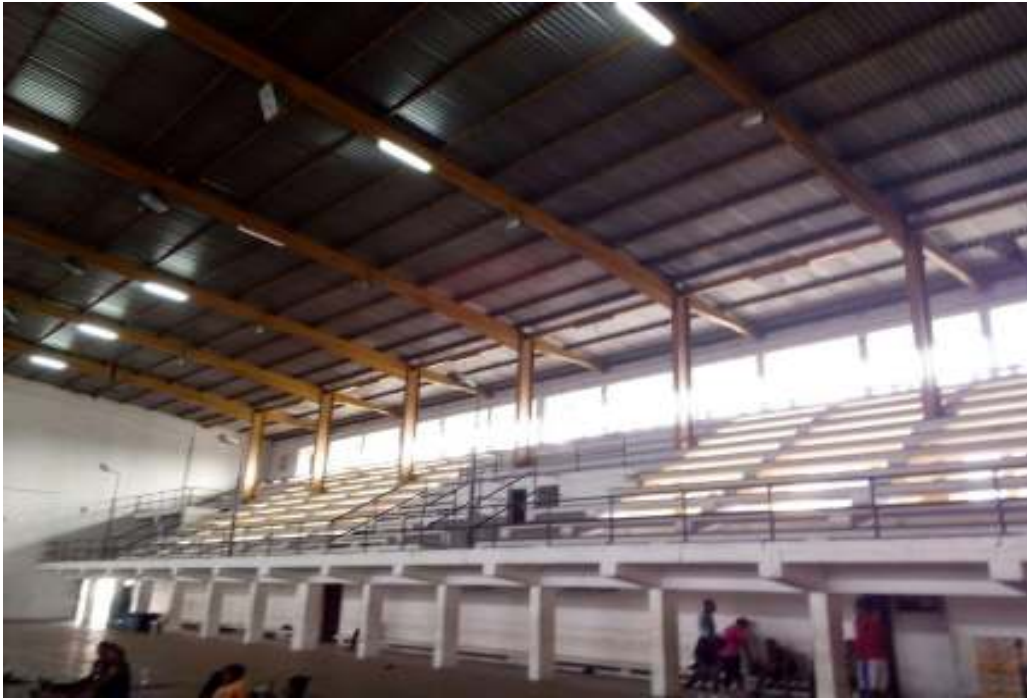
Plate 13: Showing interior of UNILAG indoor sports hall. (Source: Researchers Archive, 2015)
