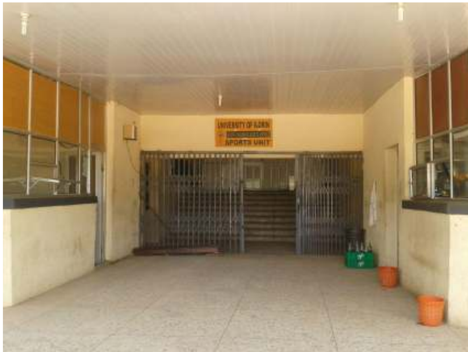
Plate 37: Showing interior (entrance area) of UNILORIN multipurpose indoor sports hall. (Source: Field Survey, 2015)
