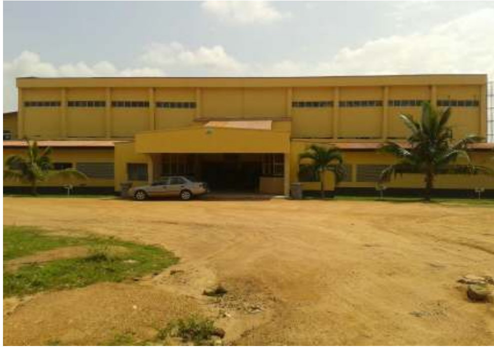
Plate 38: Showing exterior of UNILORIN multipurpose indoor sports hall. (Source: Field Survey, 2015)
