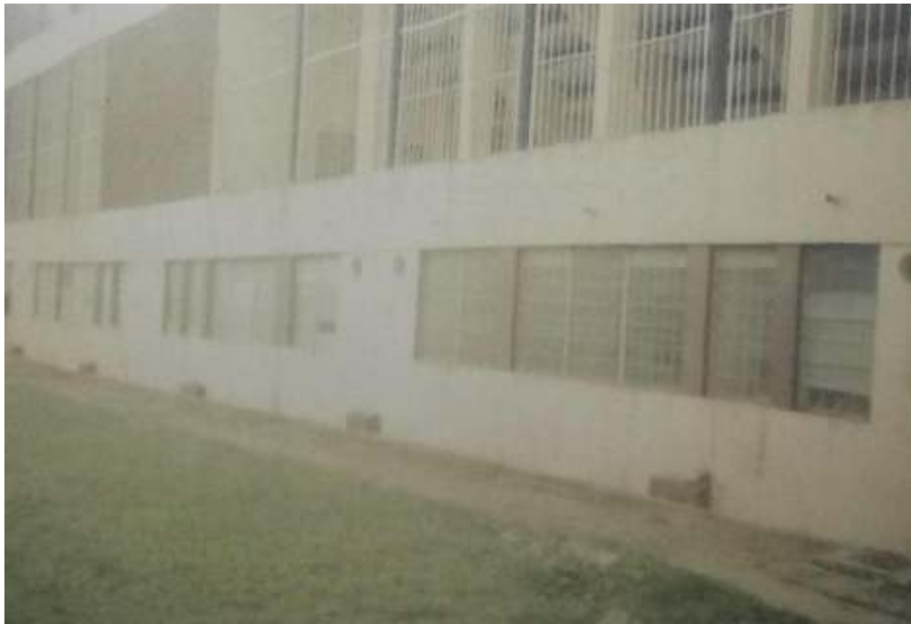
Plate 14: Showing Exterior of UNILAG indoor sports hall. (Source: Researchers Archive, 2015)
