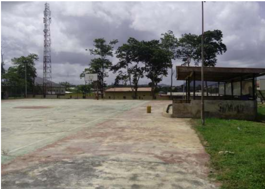
Plate 30: Showing Basketball court at FUTA sports complex. (Source: Field survey, 2015)
