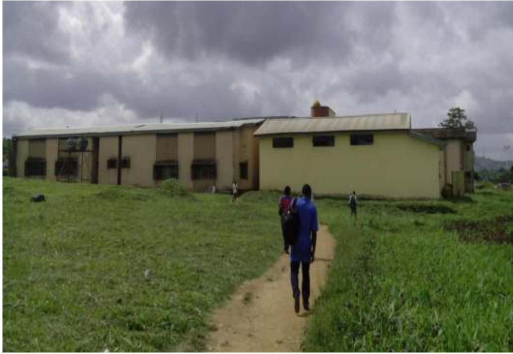
Plate 23: Showing Exterior (rear view) of FUTA indoor sports halls. (Source: Field Survey, 2015)
