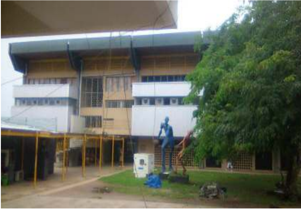
Plate 3: Showing Exterior of OAU indoor sports hall. (Source: Researchers Archive, 2015)
