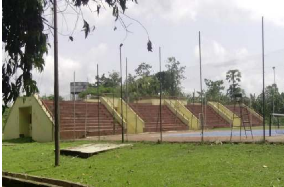
Plate 34: Showing with grandstands (without covering) for the Lawn tennis courts at FUTA sports complex. (Source: Field survey, 2015)
