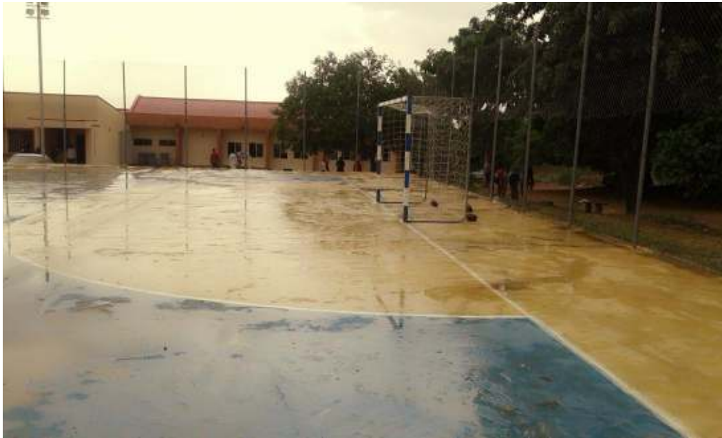
Plate 41: Showing Handball court at UNILORIN sports complex. (Source: Field survey, 2015)
