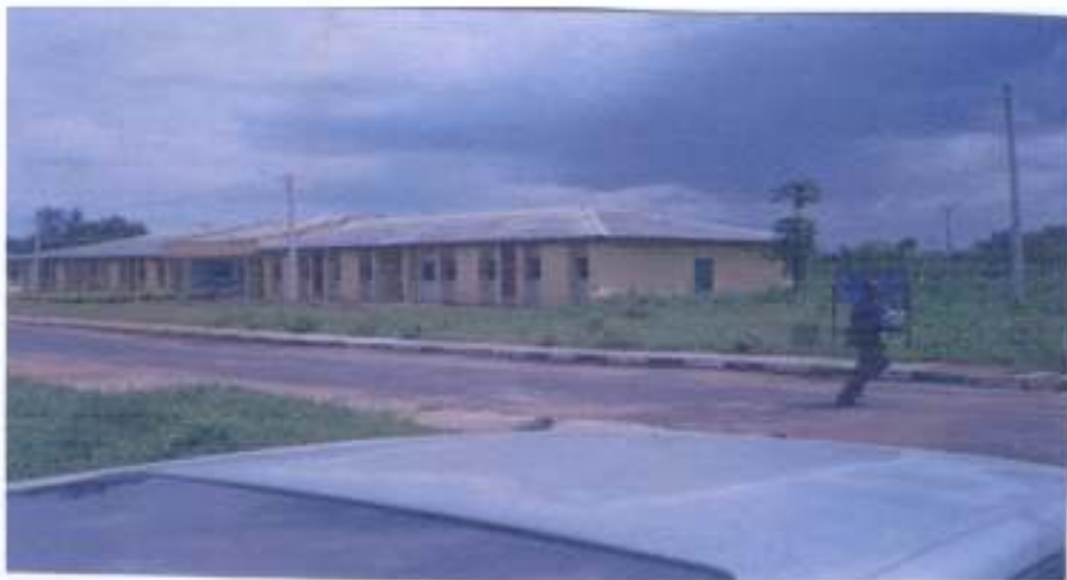
FIGURE 4.5 The present Administrative block
