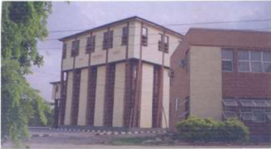
FIGURE 3.12 Showing part of the new ETF Building (UNILAG)
